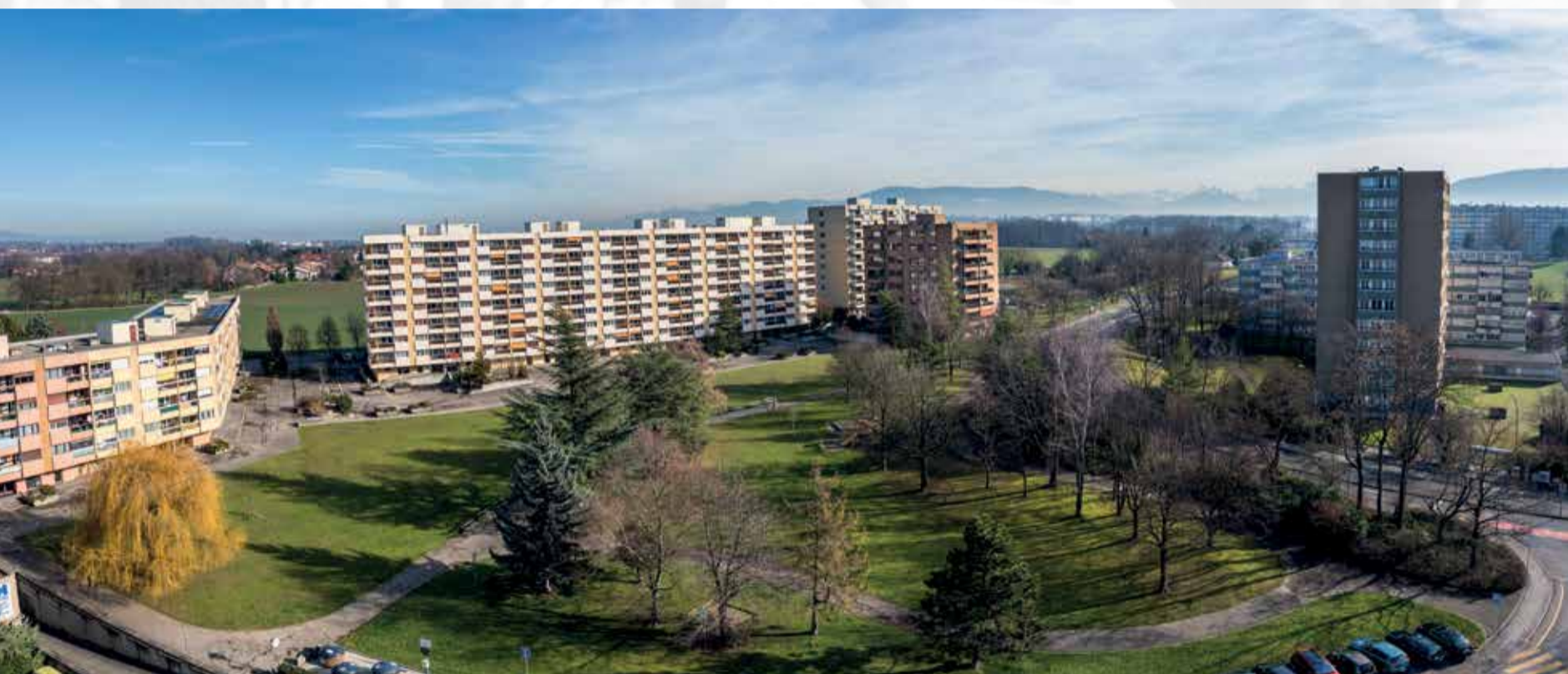
photos © Laurent Bartier
