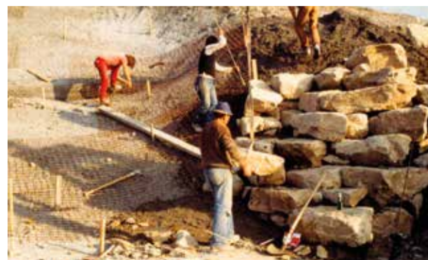
Construction du toboggan, 1988. Photo W. Kubli, ACM.
